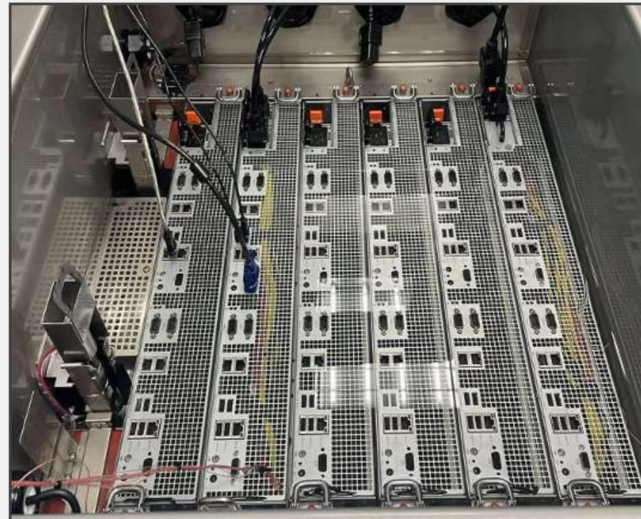
12U 15KW 浸沒式水冷槽 Fluid : Synthetic Oil (PAO Family)
